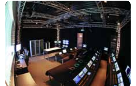
MA system stress test – to prove reliability and optimise system performance
